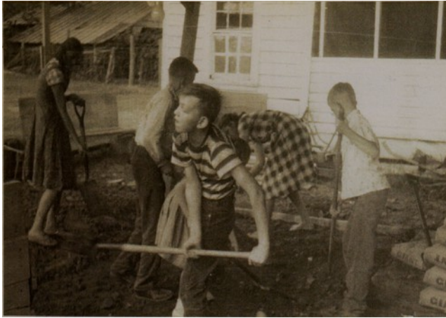
Five siblings preparing to lay concrete for the car port
